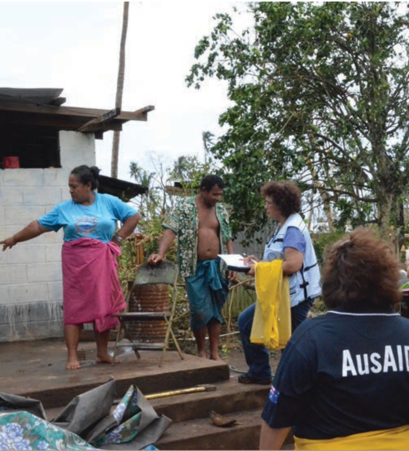
Protection concerns should be evaluated as part of needs assessments. This damage assessment was conducted following Cyclone Evan, Samoa 2012. Photo: Kevin Hadfield/AusAID
