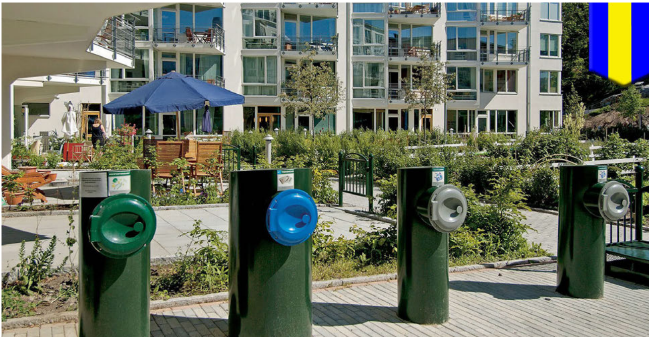
Pneumatic waste disposal technology. © TomoNews Sci and Tech
