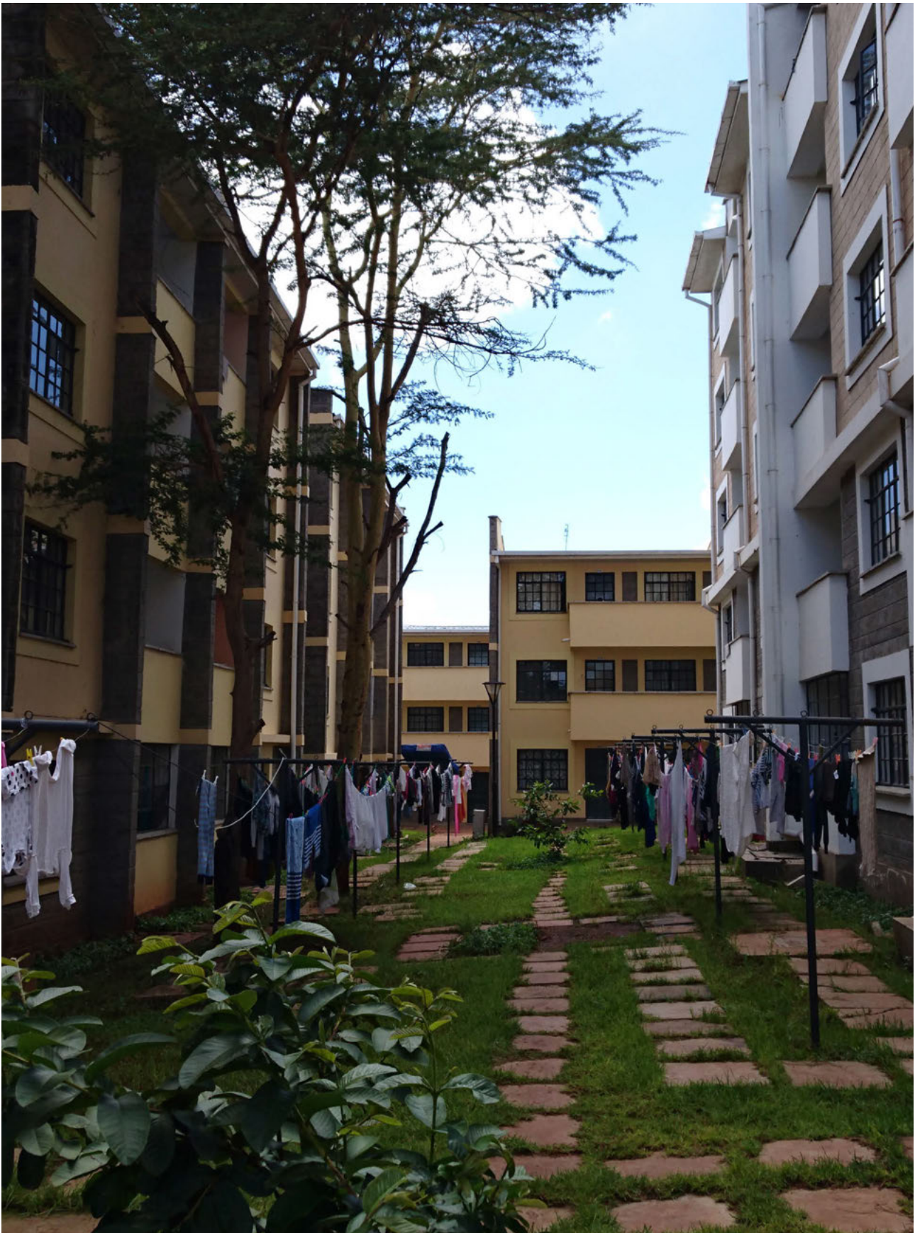
A housing project offering a variety of housing typologies with mixed density. © Baraka Mwau
