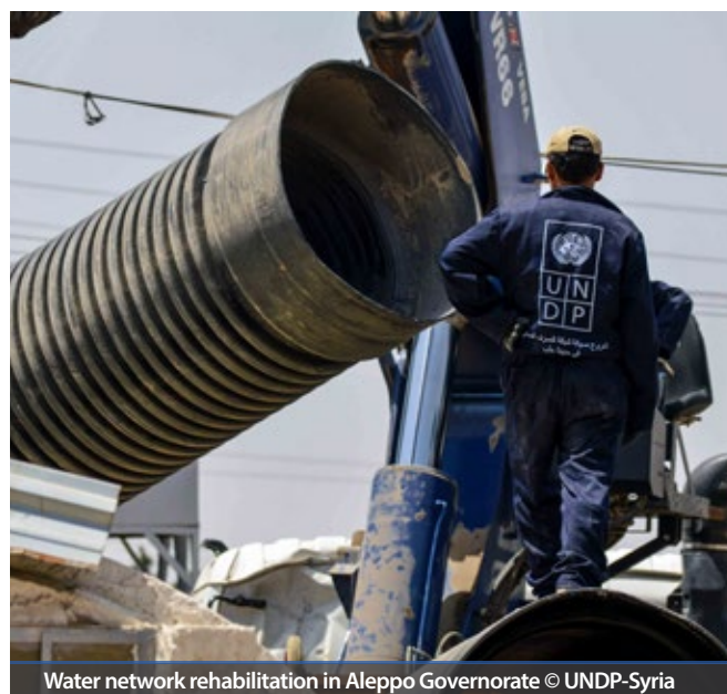
Water network rehabilitation in Aleppo Governorate © UNDP-Syria
