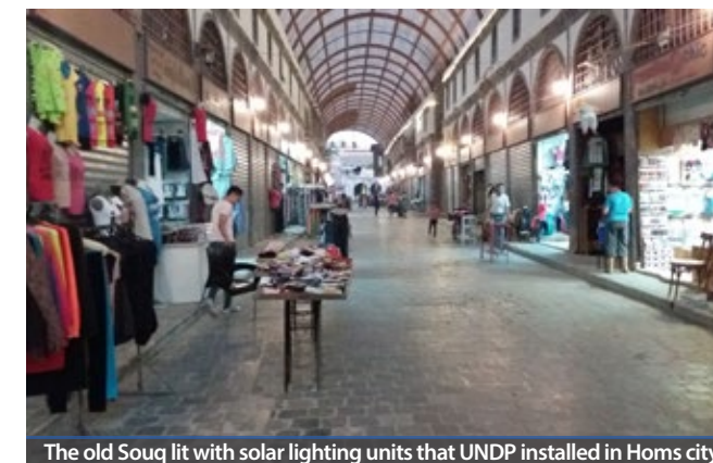
The old Souq lit with solar lighting units that UNDP installed in Homs city
